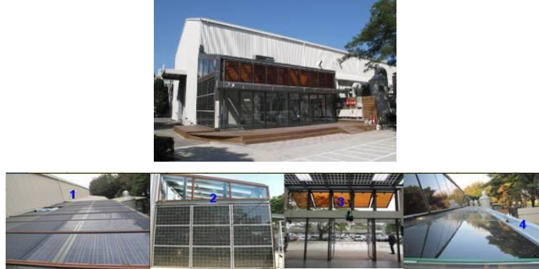
Fig. 1. The four different types of PV module were installed on different building surface.
